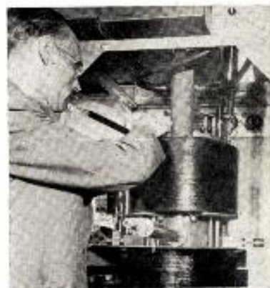
H. M. CROSBY, General Electric engineer, adjusts a new UHF velocity-modulated tube around which GE has built a 5 kw UHF television transmitter at Electronics Park, Syracuse. Transmitter will operate in the 500 mc region. GE announced the development at the IRE meeting.
